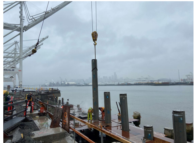
Cutting Concrete Pile
