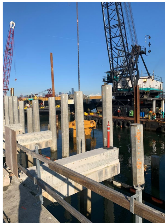
Toe Wall Pile Driving
