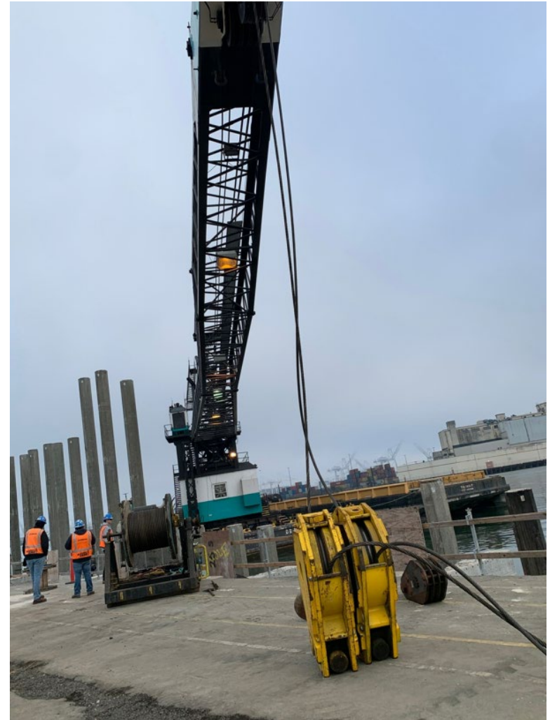
Booming Down Concrete Pile Cranes
