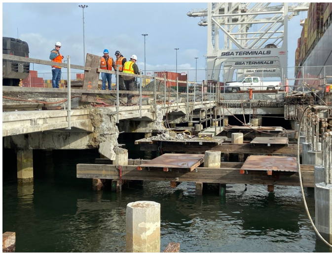
Pile doweling and Pile Cap Chipping
