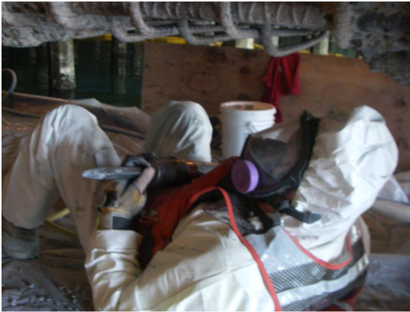
Remove Damaged Area
