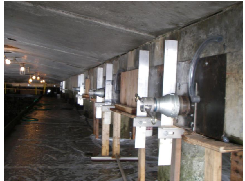
Forms Setup for Grout
