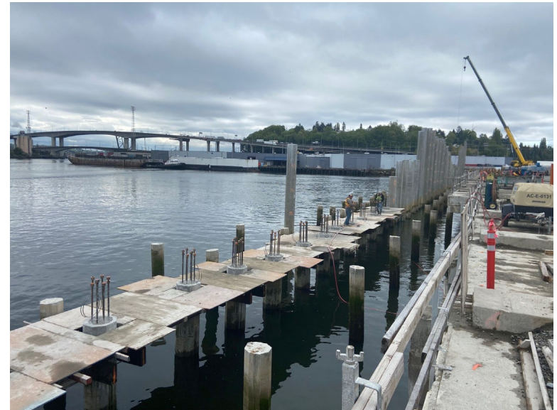
Cutting Concrete Pile
