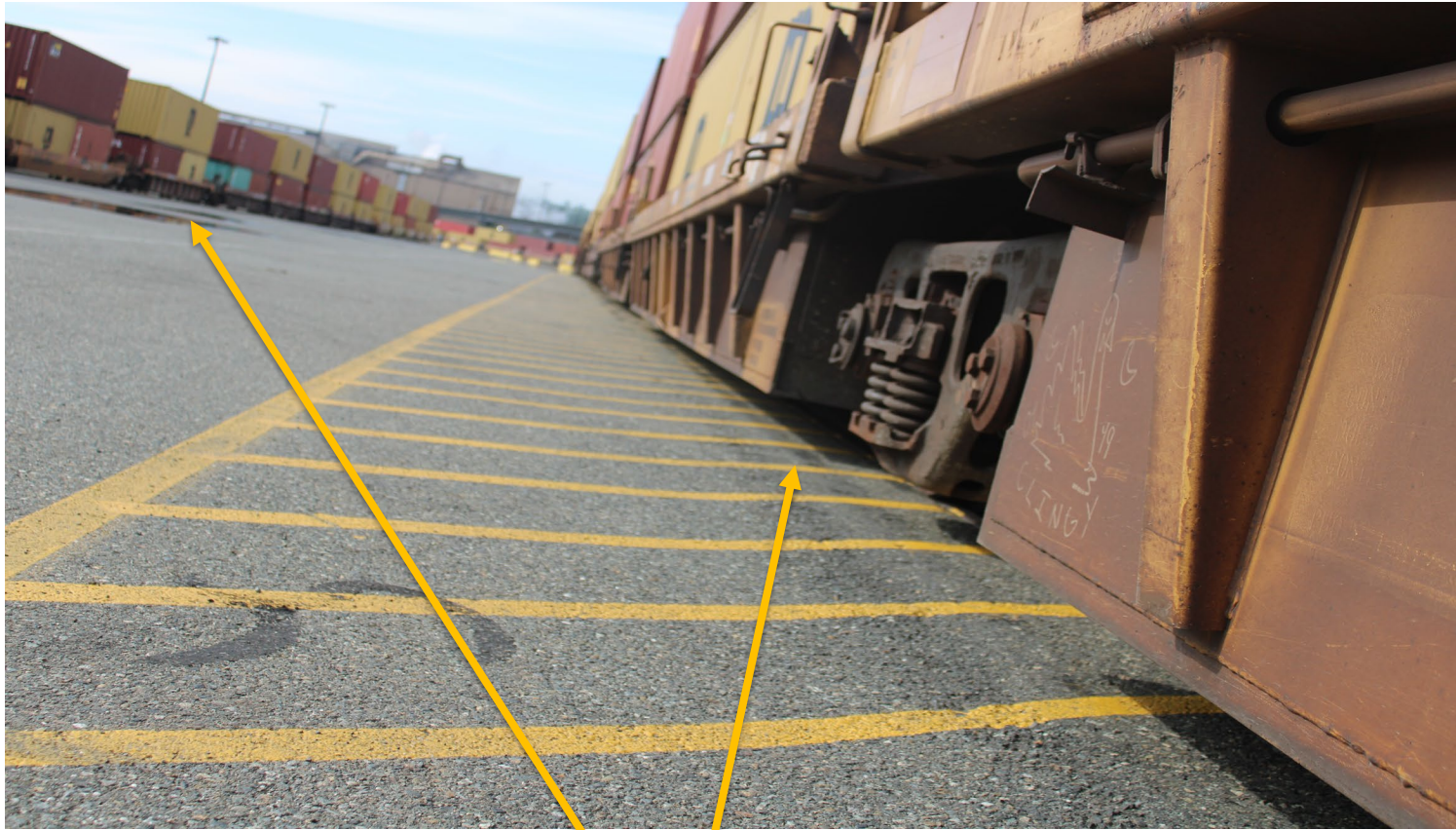
Surface deformations at edge of support structure
