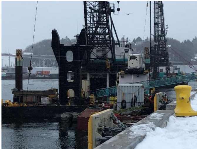
Toe Wall Pile driving
