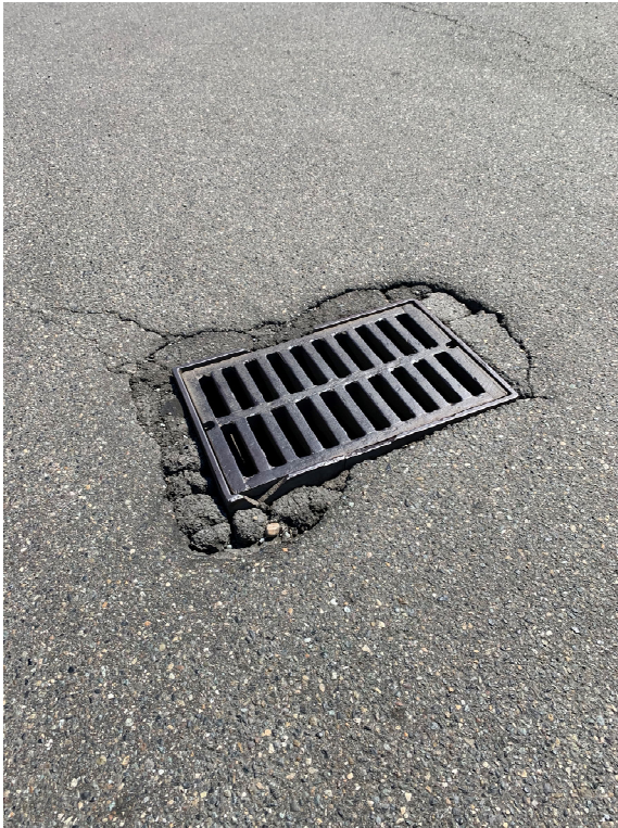
Damaged Utility Lid (Before)
