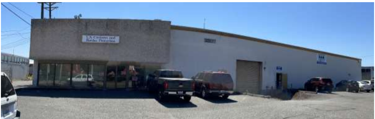
Figure 4: 2202 POT Rd Bldg.
