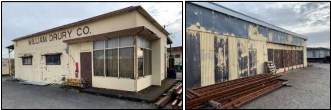
Figure 1: 2220 E 11th Bldg. (Rail Parts Storage for POT Maintenance)
