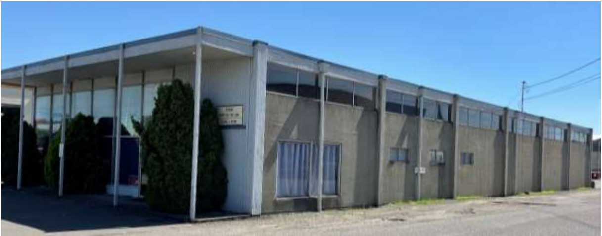
Figure 5: 2144 POT Rd Bldg.
