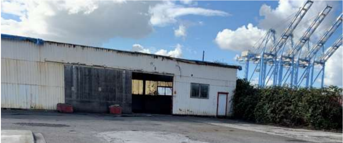
Figure 3: 1110 Alexander Bldg. (Vacant Bldg. South of TOTE Terminal)
